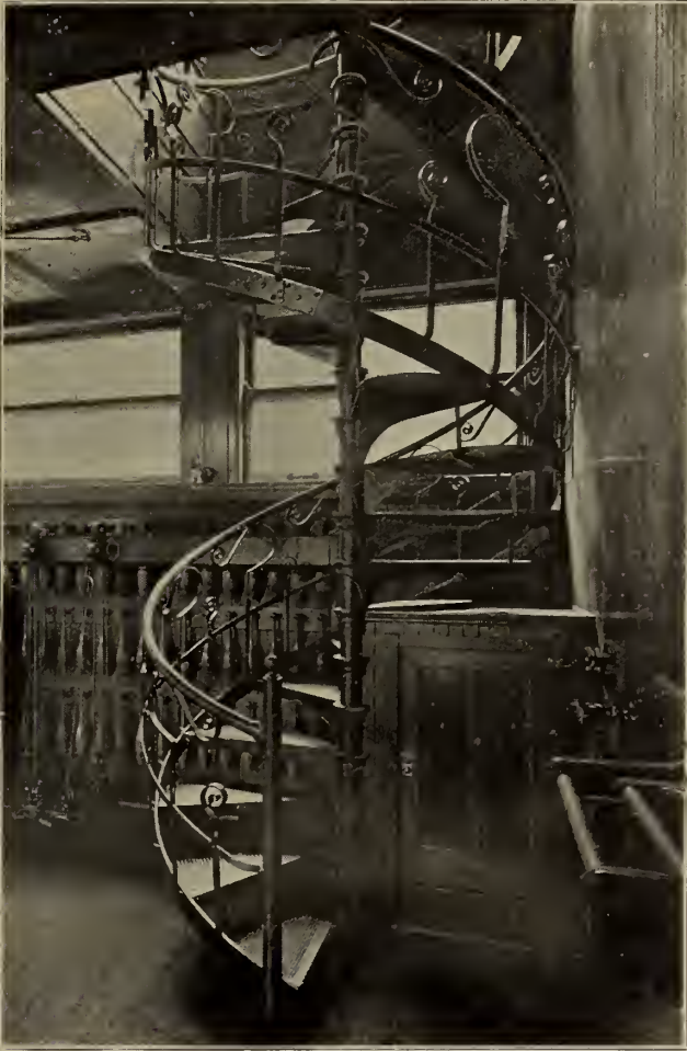
A.—SPIRAL STAIRWAY, ASSOCIATION BUILDING, CHICAGO. Wrought Iron, Bower-Barffed.
